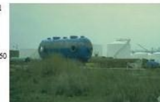
Above ground storage tanks
